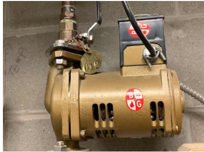
Hot Water Storage Tank, DHW Circulation Pump, and Unit Label
