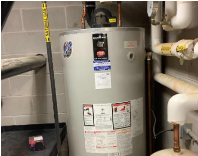
Hot Water Storage Tank, DHW Circulation Pump, and Unit Label
