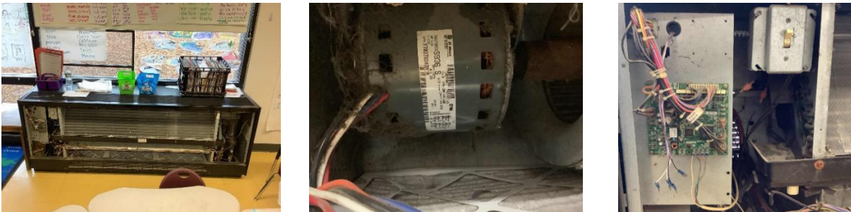
Unit Ventilator, Supply Fan Motor, and Electronic Controls
