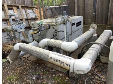
Hot Water Boiler and Circulation Pump
