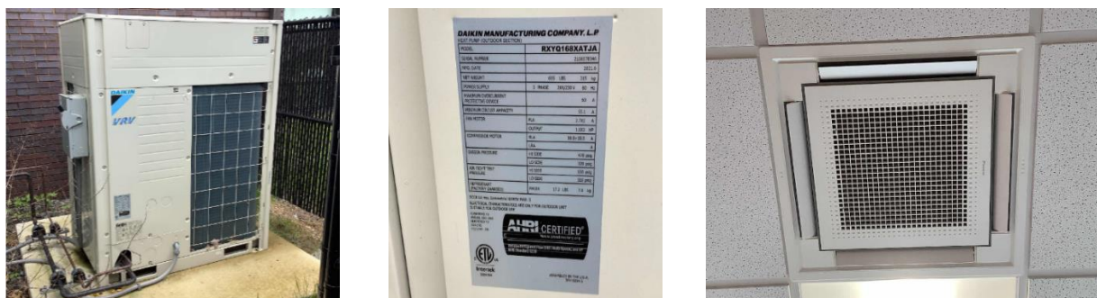
Outdoor Condensing Unit, Unit Label, and Indoor Evaporator
