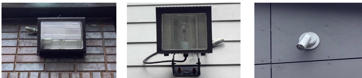
Wall Pack, Flood, and Spot Light Fixtures
