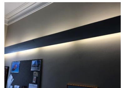
Wall Mount Linear Fluorescent Fixture
