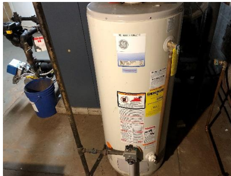
Storage Tank Water Heater
