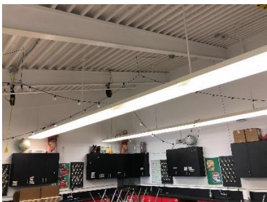
Classroom Pendant and Surface Mount Linear Fluorescent Fixtures
