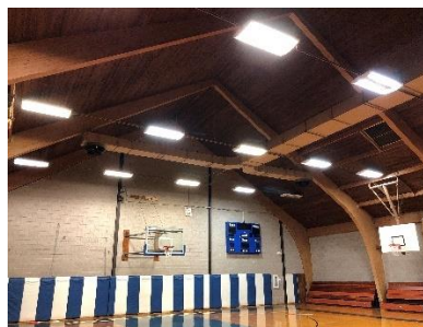
Linear Fluorescent Pendant Mount Fixtures
