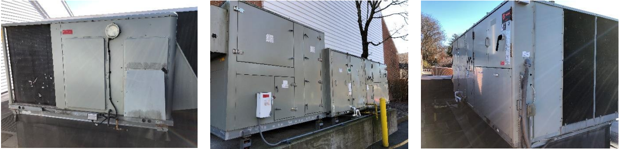
Packaged Roof Top Units (RTUs)
