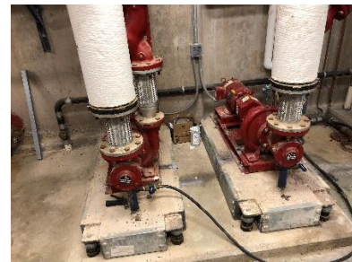
Heating Hot Water Pumps
