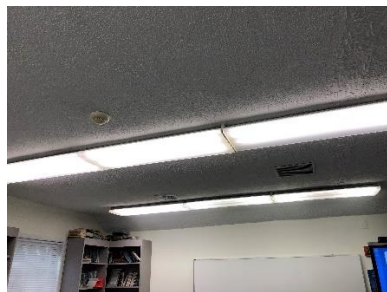
Classroom Pendant and Surface Mount Linear Fluorescent Fixtures
