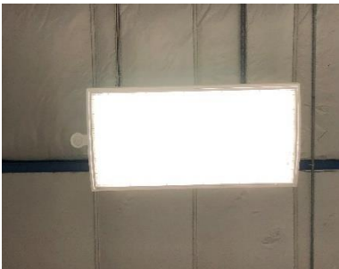
Pendent Mount Troffer Fluorescent Fixture
