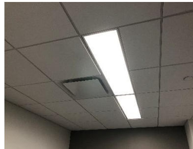
Recessed Troffer Fluorescent Fixture
