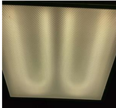
2-Foot Long T8, U-Shape Fluorescent & LED Fixtures
