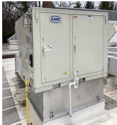
Package roof top units (RTUs)
