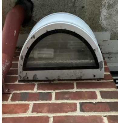
LED Wall Mounted Fixtures
