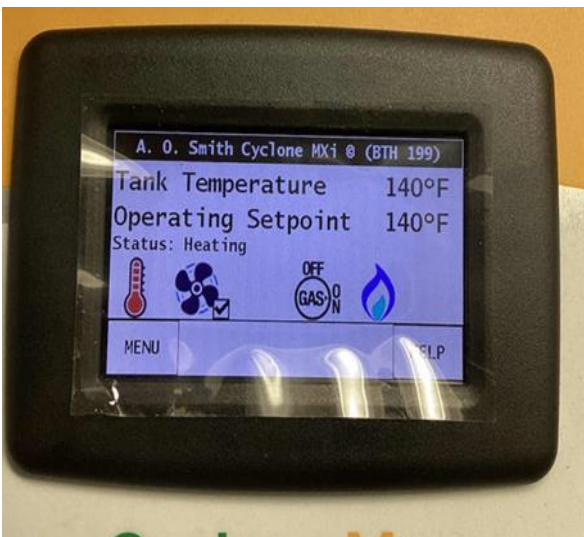
Touch Screen (Condensing Water Heater) & Booster Water Heater
