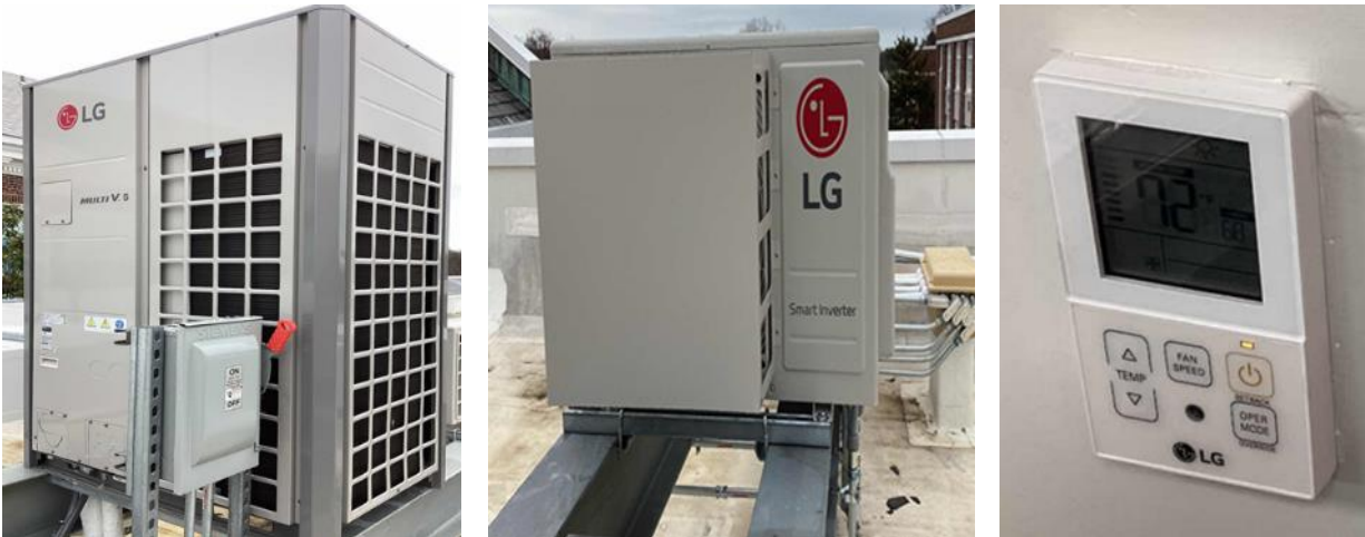
Media Center Heat Pumps & Programmable Thermostat
