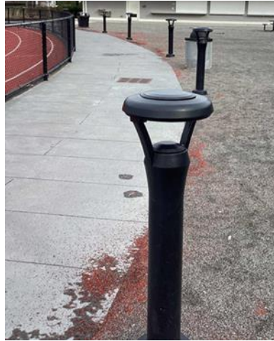
Pole Fixture w/ LED Corn Bulb & LED pole fixtures
