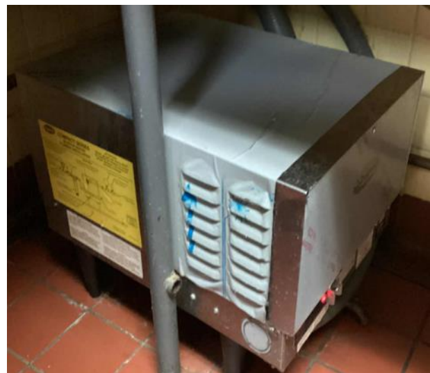
Touch Screen (Condensing Water Heater) & Booster Water Heater
