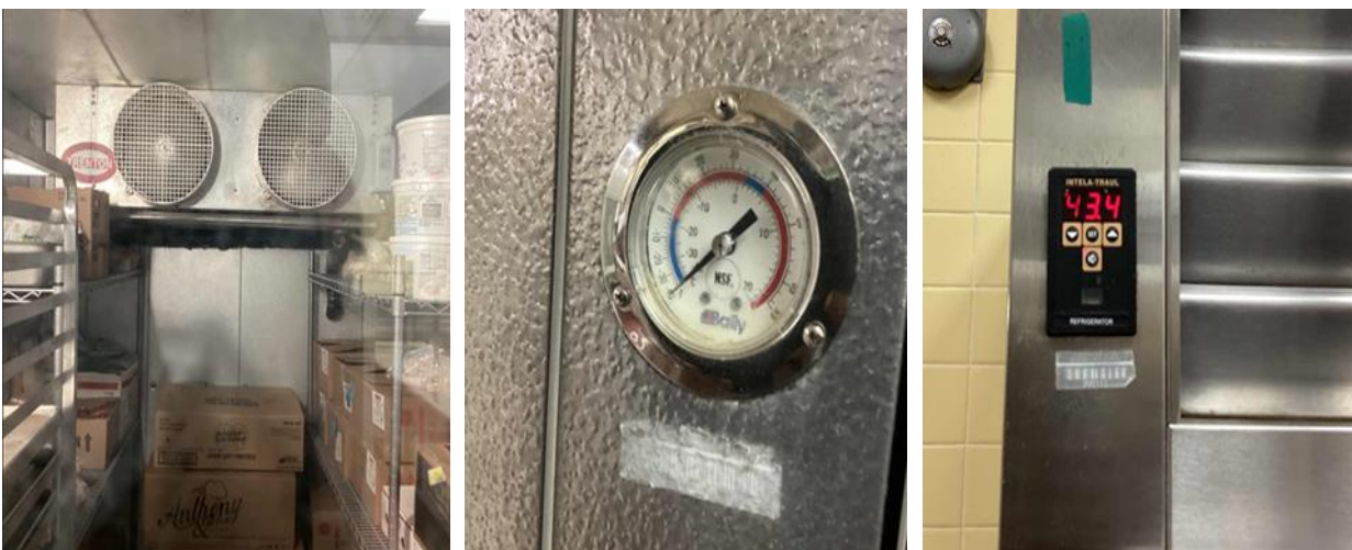
Evaporator fans, freezer & refrigerator temperatures
