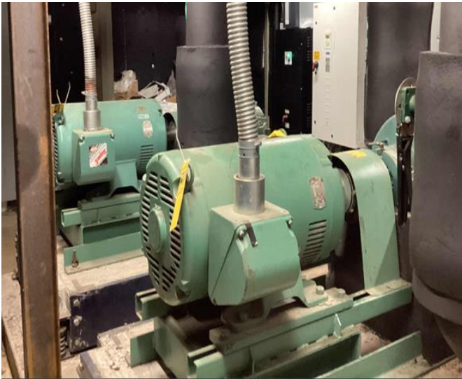
Variable Flow Condenser Water Pumps
