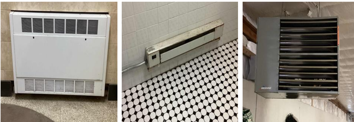
Electric resistance heaters
