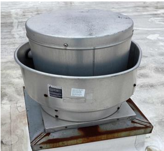
General exhaust fan & Classroom Fume Hood (EF-1).
