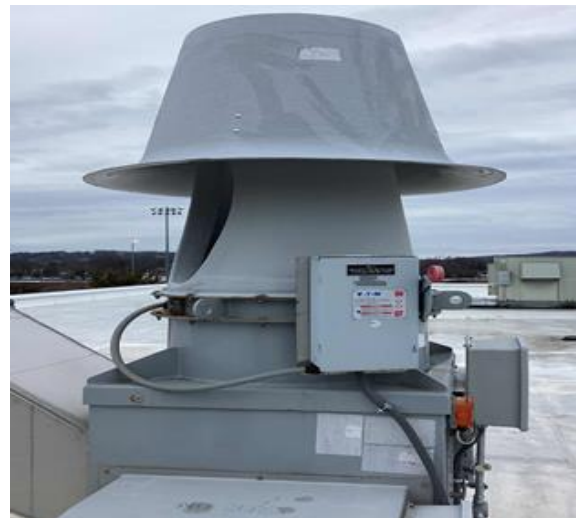
General exhaust fan & Classroom Fume Hood (EF-1).
