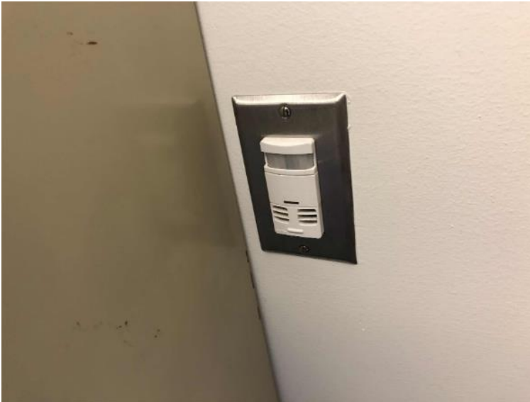
Wall Switch Sensors
