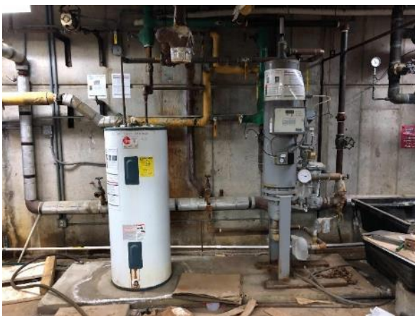
Storage Tank Water Heater
