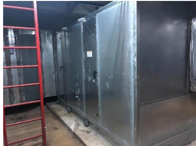
Air Handling Unit (AHU)
