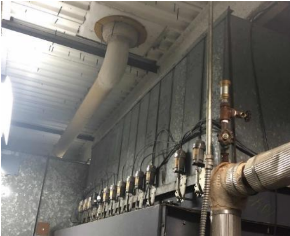
Air Handling Unit (AHU)
