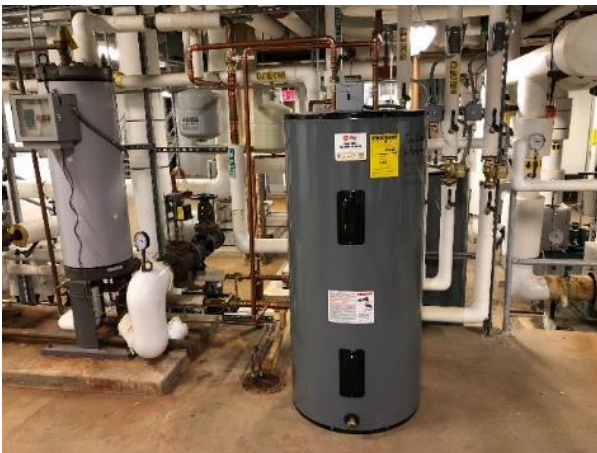
Hot Water Storage Tank
