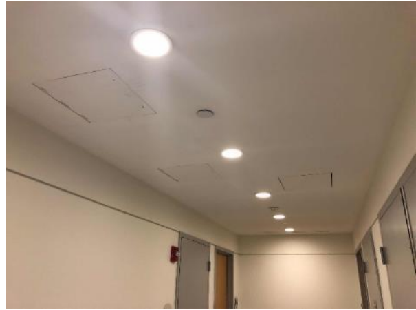
Recessed Can Fixtures
