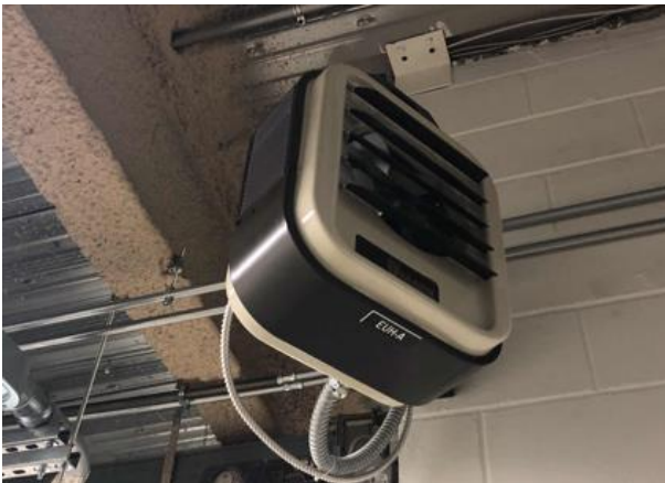
Electric Resistance Heater
