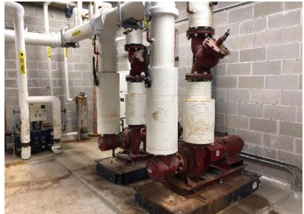
Heating Hot Water Pumps
