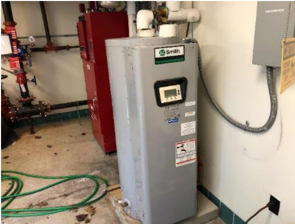
Storage Tank Water Heater
