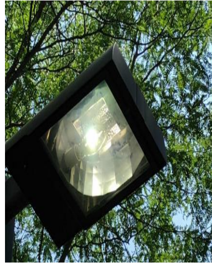
Exterior Metal Halide Fixture
