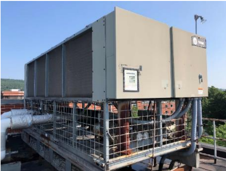
Air Cooled Screw Chiller
