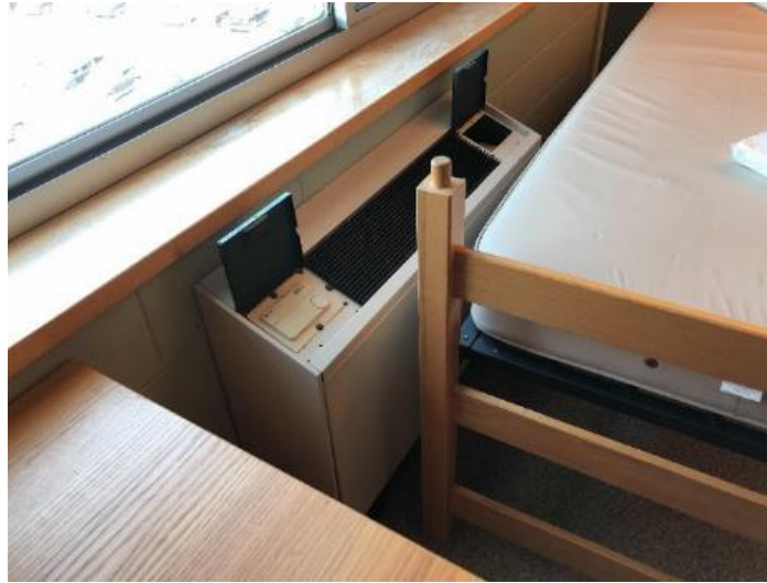
Residential Fan Coil Unit – with Hot Water and Chilled Water Coils
