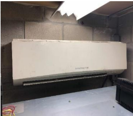
Elevator Room AC Unit
