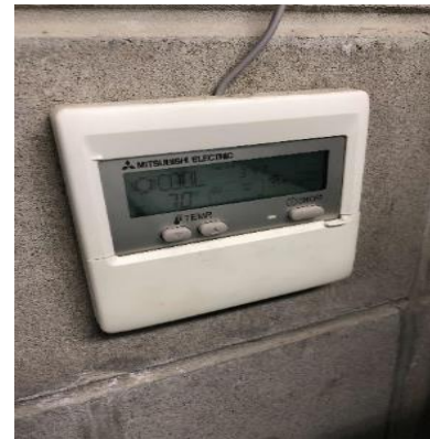
Programmable Thermostat
