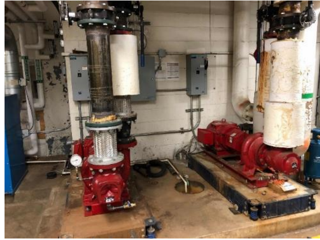
Heating Hot Water Pumps
