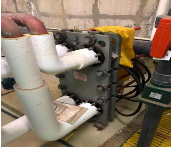
Heat Exchanger
