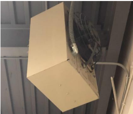
Electric Resistance Heaters
