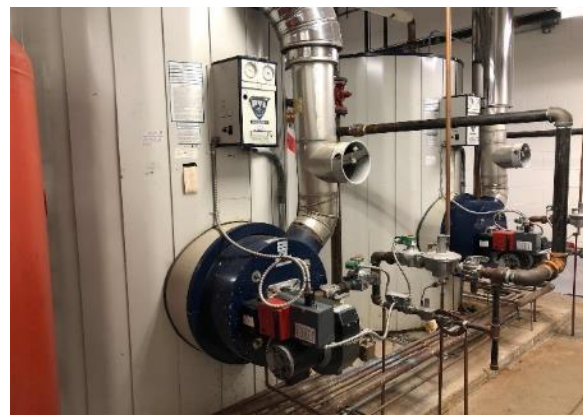
Hot Water Storage Water Heaters
