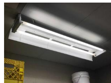
Surface Mount Linear Fluorescent Fixtures
