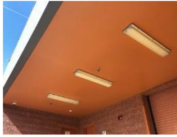
Linear Fluorescent Canopy Fixtures
