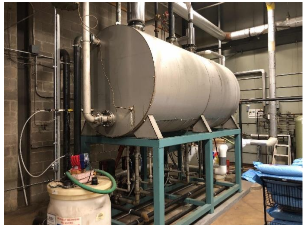
Steam Boilers and Condensate Return
