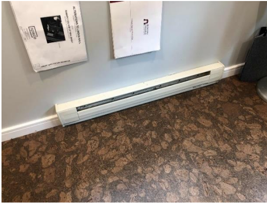
Electric Resistance Heat
