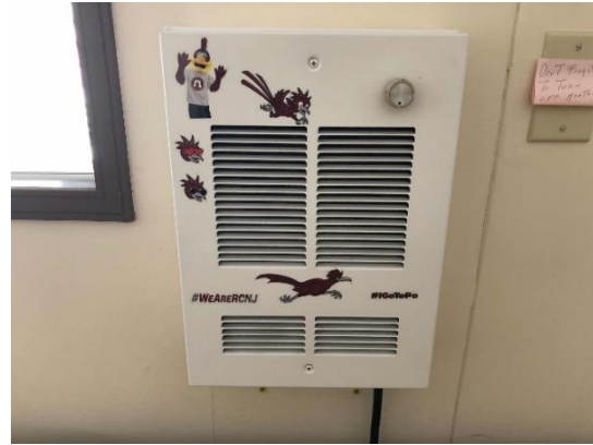
Electric Resistance Heat
