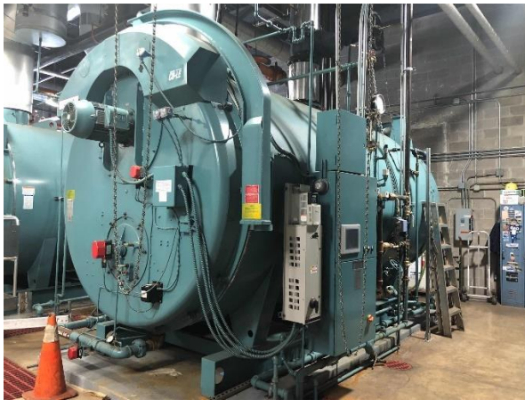
Steam Boilers and Condensate Return
