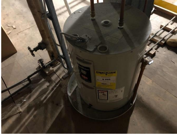
Hot Water Storage Heater
