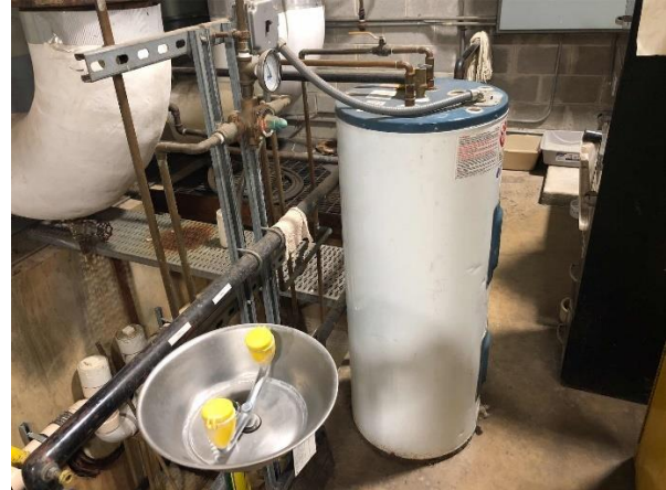
Hot Water Storage Heater
