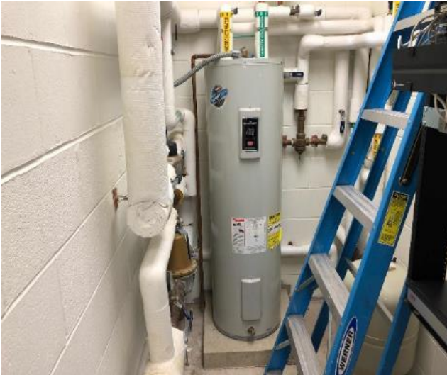
Hot Water Storage Heater
