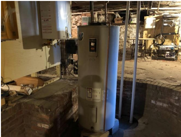
Electric Storage Water Heater
