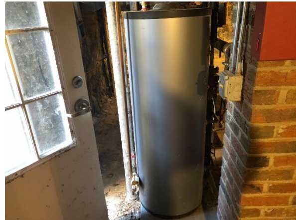
Natural Gas-fired Indirect Water Heater
