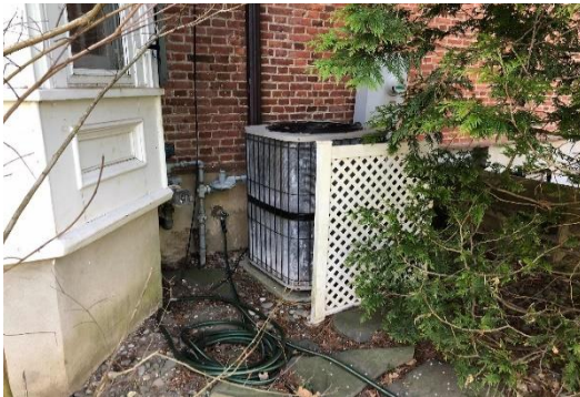
Cooling Condensing Unit
