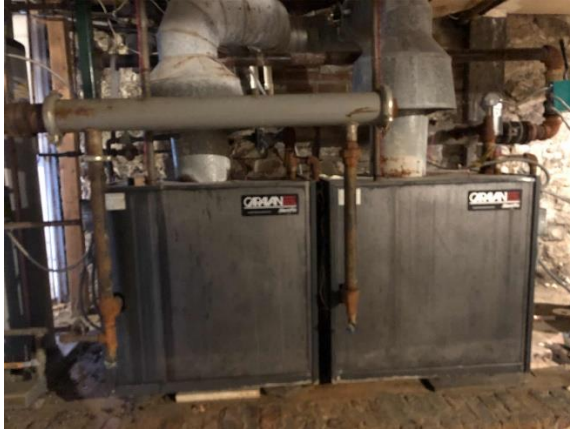
Non-condensing Water Boilers
