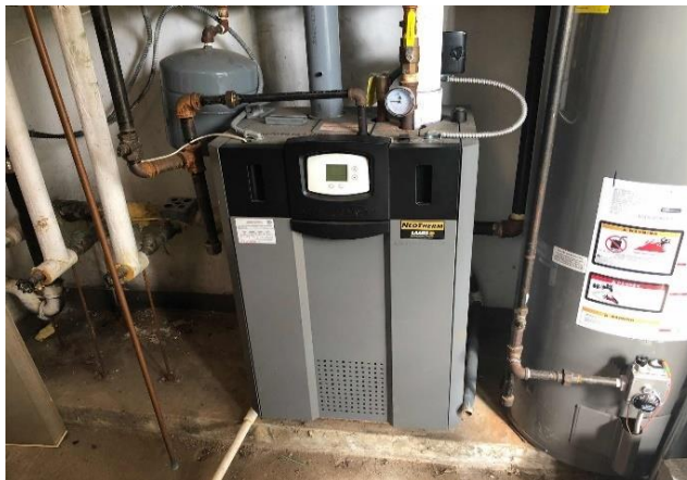
Condensing Hot Water Boiler
