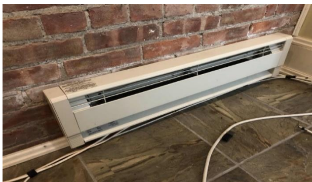
Havemeyer House – Electric Resistance Heater
