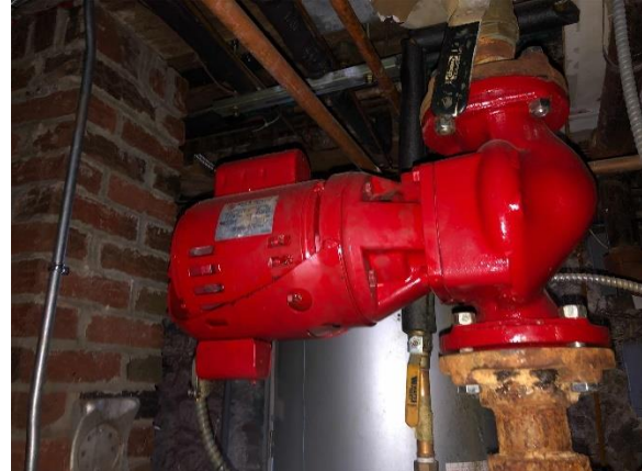
Heating Hot Water Pumps
