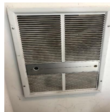
Health Services – Electric Resistance Heater
