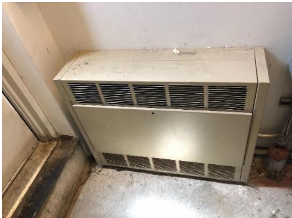
Electric Resistance Heaters
