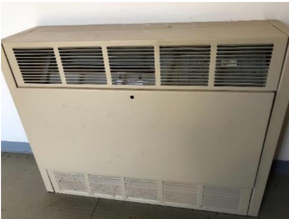
Electric Resistance Heaters
