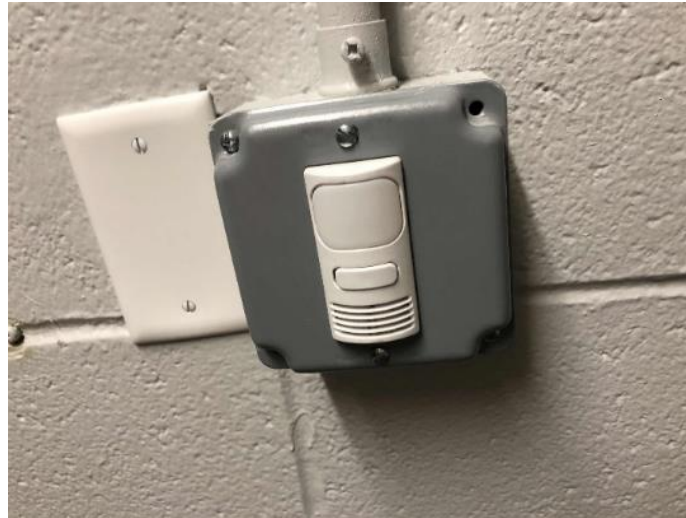
Wall Switch Occupancy Sensor
