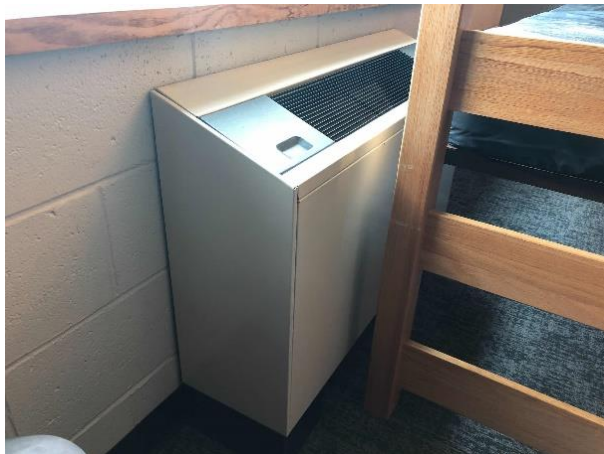
Residential Fan Coil Unit – With Hot Water and Chilled Water Coils
