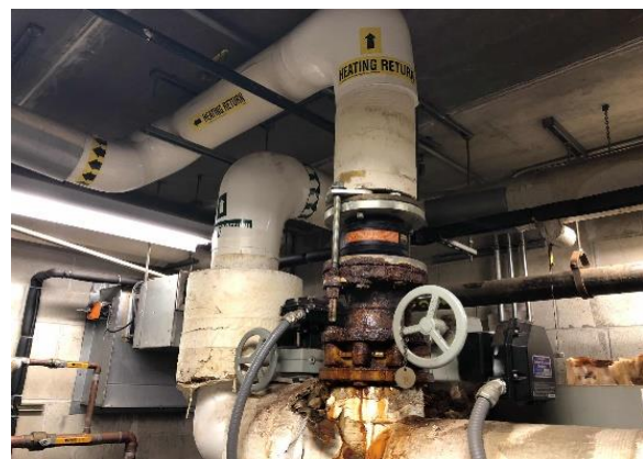
Dual Temperature Heat Exchanger
