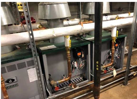
Non-condensing Hot Water Boilers
