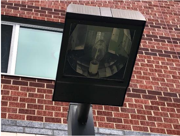
Exterior Metal Halide Fixtures
