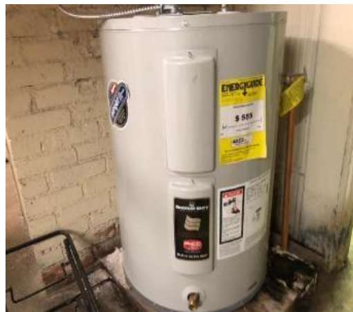
Hot Water Storage Tank
