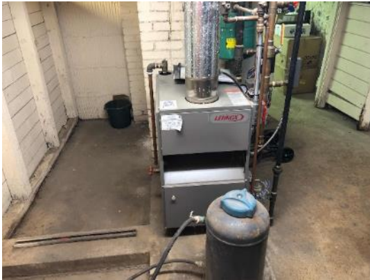
Hot Water Boiler
