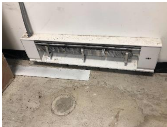
Electric Resistance Heater
