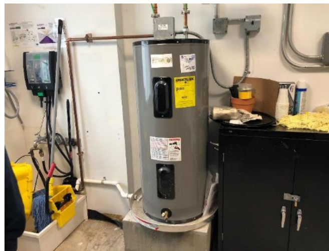
Domestic Hot Water Storage Heater
