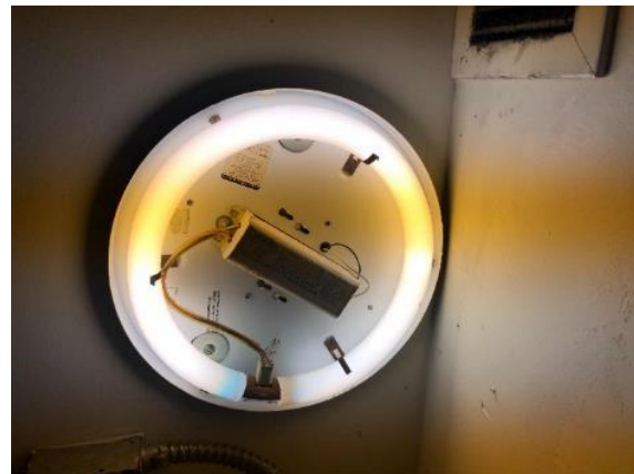
Circline Fluorescent Light Fixture
