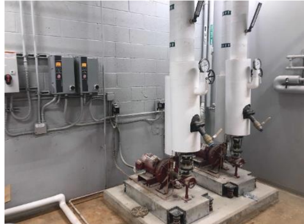
Heating Hot Water Pumps
