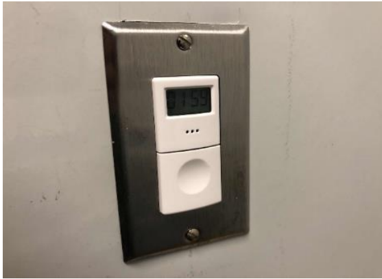
Wall Switch Sensor
