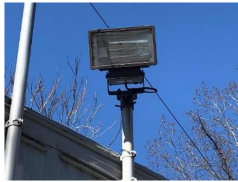
Sculpture Studios – Northeast – Exterior 250-watt HPS fixture
