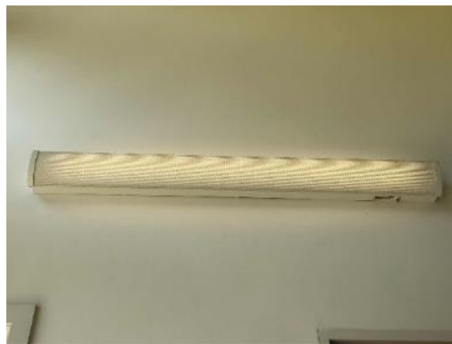
Restroom 2-foot T5 HO fixture
