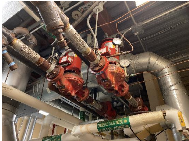
Heating Hot Water Pumps
