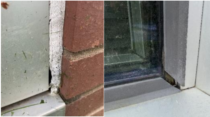
Poor Window Seal Conditions
