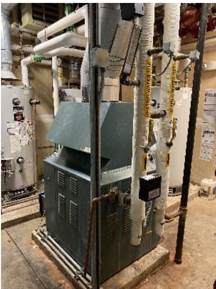
Raypak Hydronic Boiler
