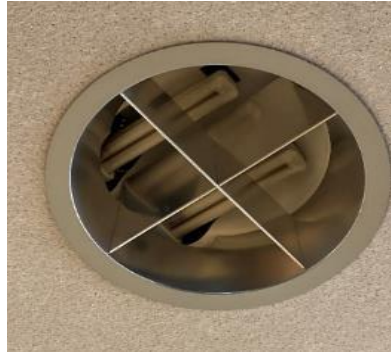
2-Lamp Recessed Canned CFL Fixture
