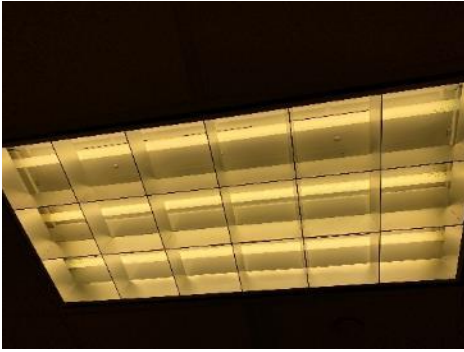
3-Lamp 4-foot T8 Recessed Parabolic Fixture
