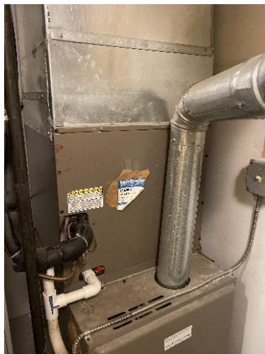
AHU and Furnace
