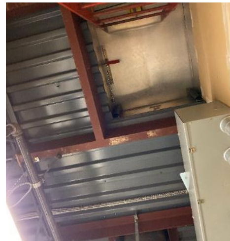
Exposed Steel Construction Ceiling in Mechanical Room
