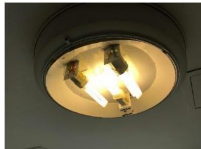
Plug-in CFL Fixture
