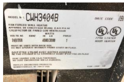
Electric Resistance Heaters
