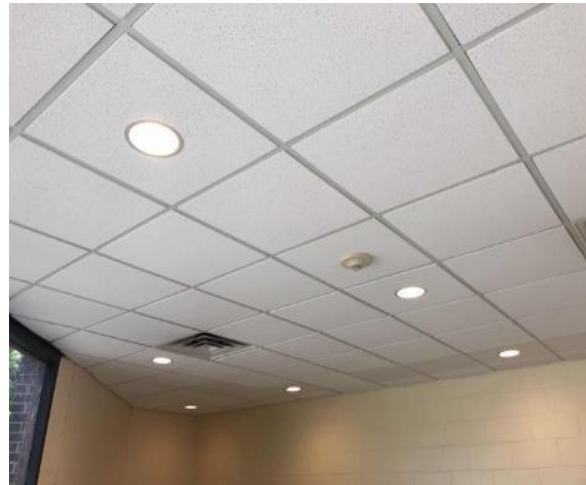
Recessed Can Fixtures
