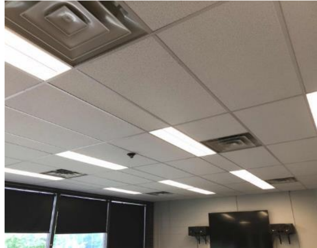
Linear Fluorescent Light Fixtures
