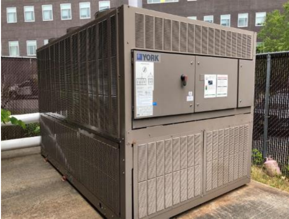
Air Cooled Scroll Chiller
