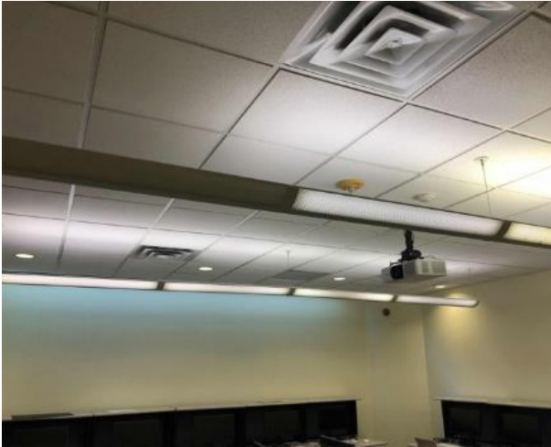
Linear Fluorescent Light Fixtures
