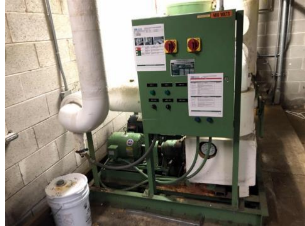
Air Cooled Scroll Chiller
