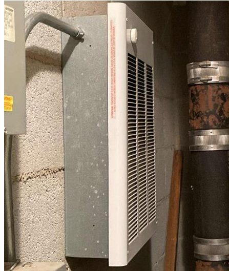
Comfort Station East Electric Resistance Heater
