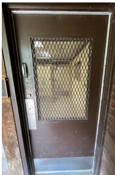
Comfort Station East: Metal Doors with Wire Windows & Solid Metal Doors
