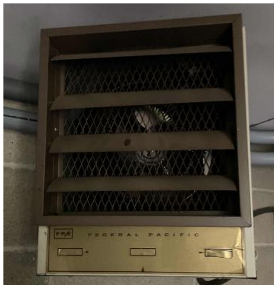
Generator Building Electric Resistance Heater
