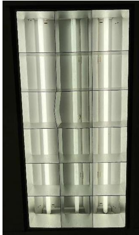
Comfort Station North 4-Foot T8 Linear Fluorescent Lights
