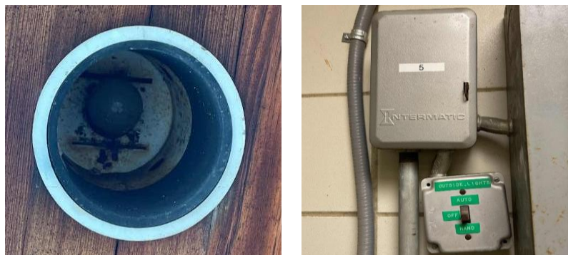
Incandescent Recessed Can Fixture & Timeclock w/ Optional Manual Control Switch
