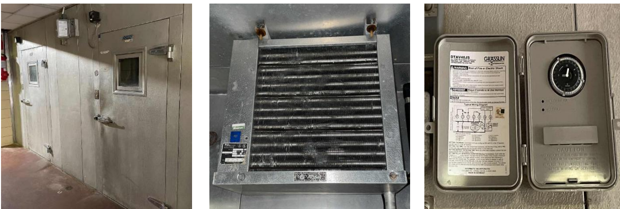
Walk-In Freezer, Evaporator, & Defrost Control
