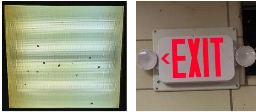
Linear Fluorescent T12 Lamps & LED Exit Sign
