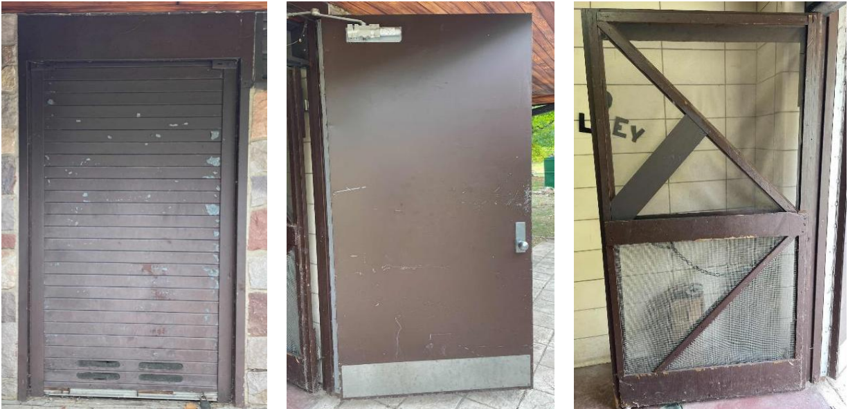
Roll Up Metal Door, Hollow Metal Door, & Wood Framed Screen Door
