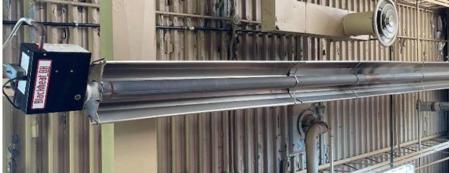
Propane-Fired Infrared Heater
