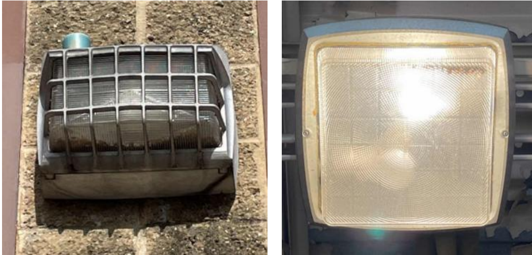
Exterior HPS Wall Pack & Ceiling Mounted Fixture W/ A19 LED
