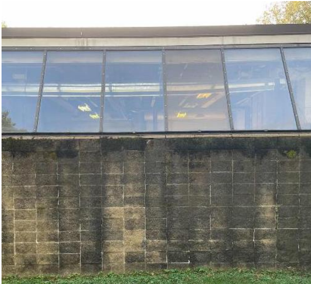
Facility Fixed Single Pane Skylights & Operable Double Paned Windows
