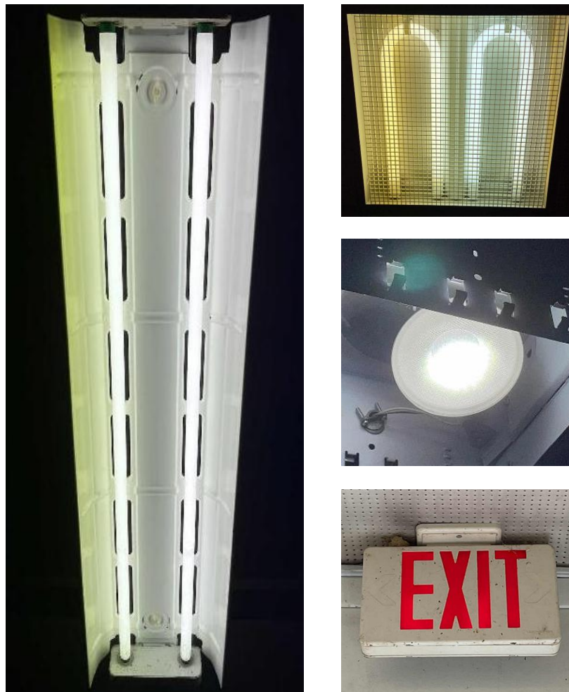
Linear Fluorescent T8 Lamps, U-Bend T12 Lamps, LED Par20 Lamp, & LED Exit Sign
