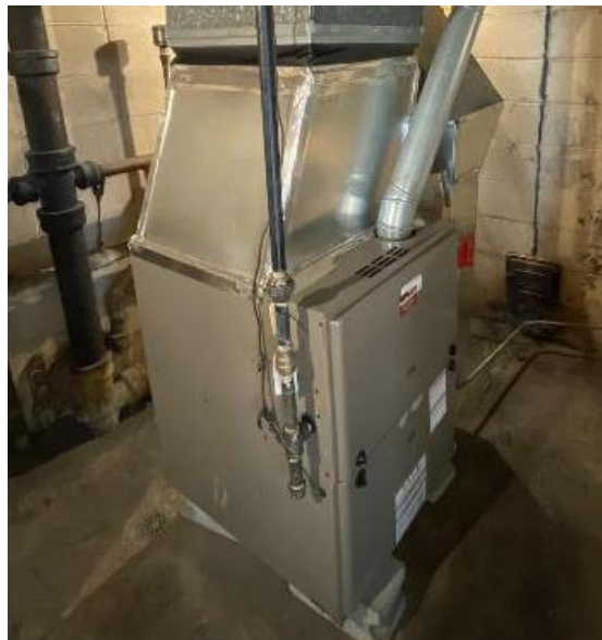
Propane-Fired Forced Air Furnace
