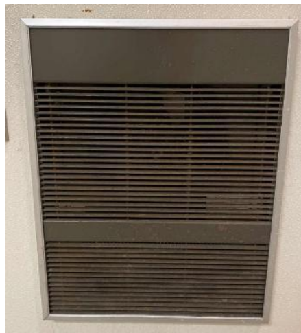
Wallace Interpretive Center Public Restrooms Electric Resistance Heater
