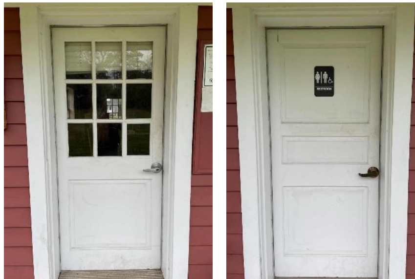
Wood Door w/ Glass Lite & Solid Wood Door
