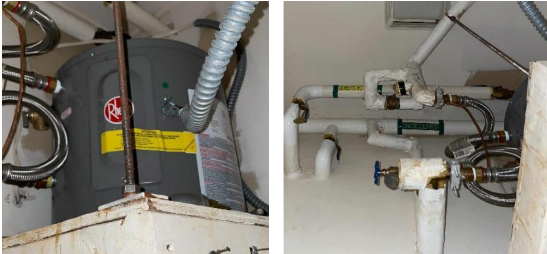
Wallace Interpretive Center DHW Tank & DHW Pipe Insulation
