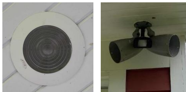
Recessed Can w/ Biaxial CFL Lamps & Halogen Flood Lights
