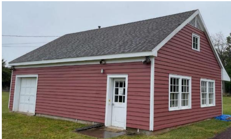
Building Envelope w/ Wood Clapboard Siding
