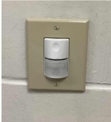
Wall Mounted Occupancy Sensors
