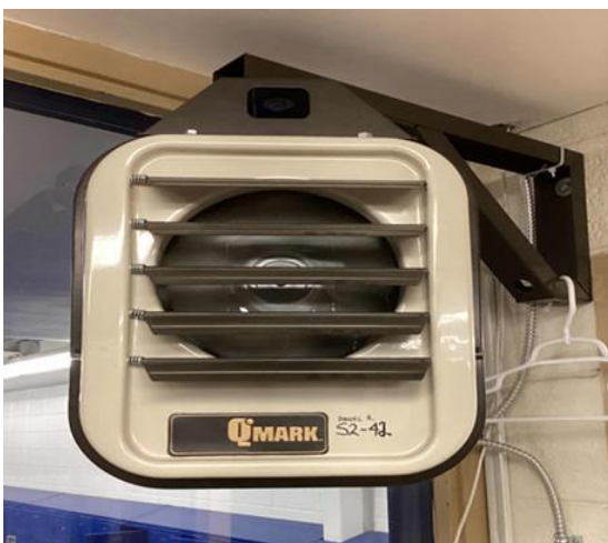
High School Electric Resistance Heaters
