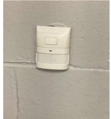
Wall Mounted Occupancy Sensors
