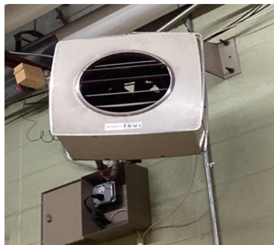
High School Electric Resistance Heaters
