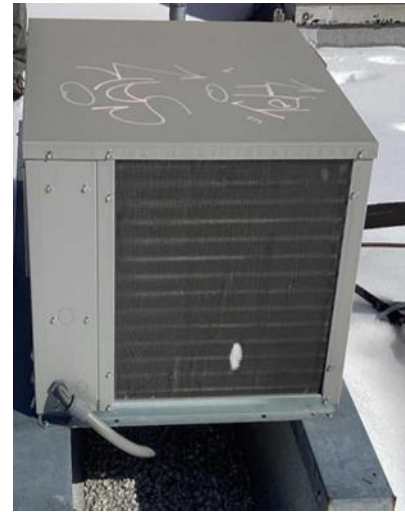
Walk-in Condensing Box
