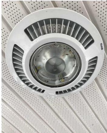
Exterior LED Ceiling Mounted Fixtures
