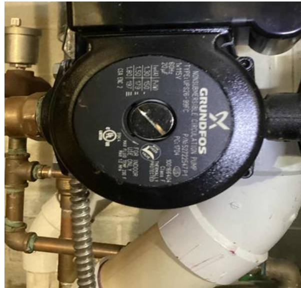
Fractional Circulating Pumps
