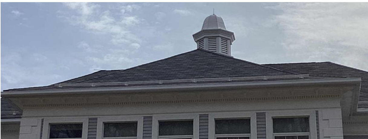
Pitched Roof w/ Asphalt Shingles
