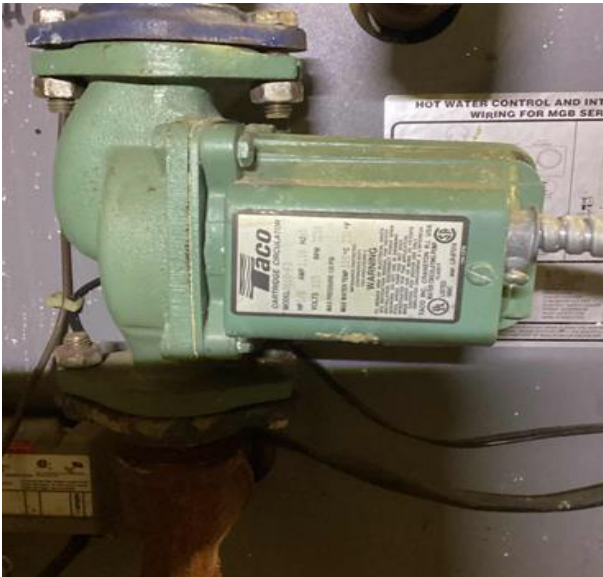
Fractional Circulating Pumps
