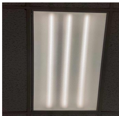
4 Foot LED Linear Tubes
