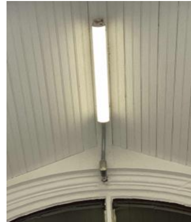
Exterior LED Ceiling Mounted Fixtures
