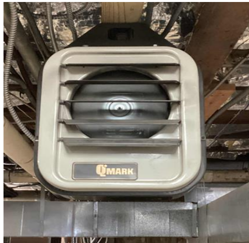
Electric Resistance Heater
