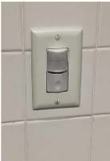
Wall Mounted Occupancy Sensor
