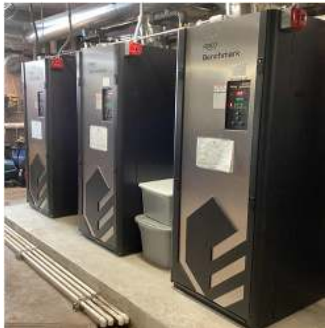
Condensing Boilers
