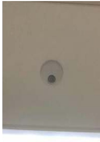
Ceiling Mounted Occupancy Sensor
