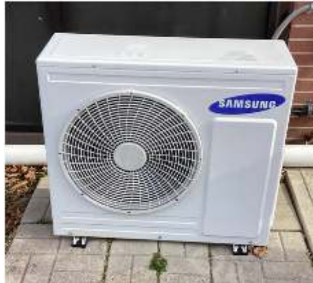
Mini Split Heat Pump –Outdoor Condensing Unit
