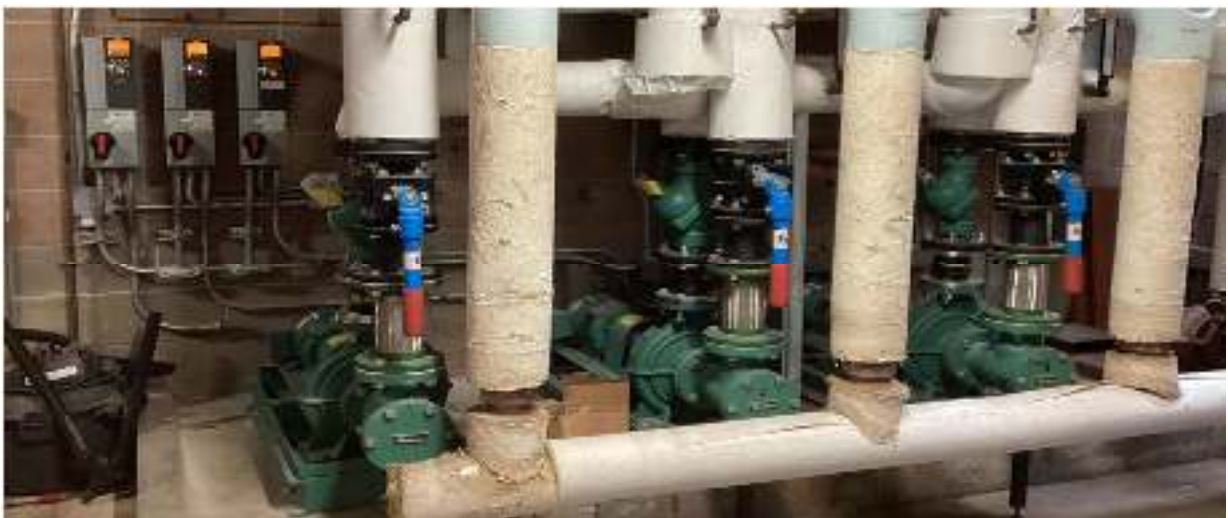
3 hp Hot Water Pumps with VFDs
