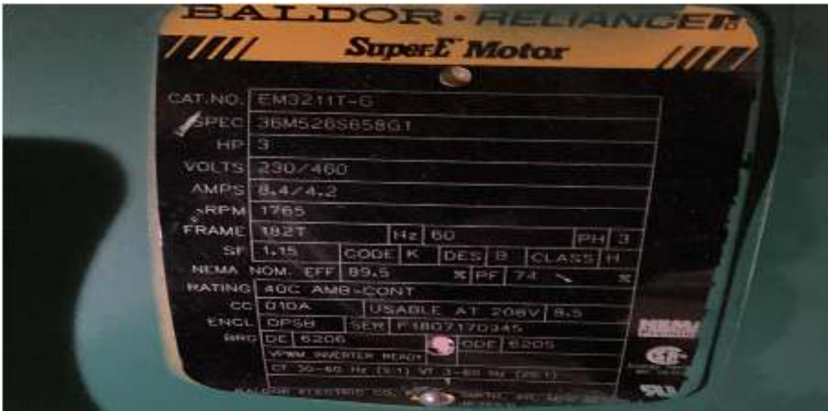
3 hp Hot Water Pump Tag
