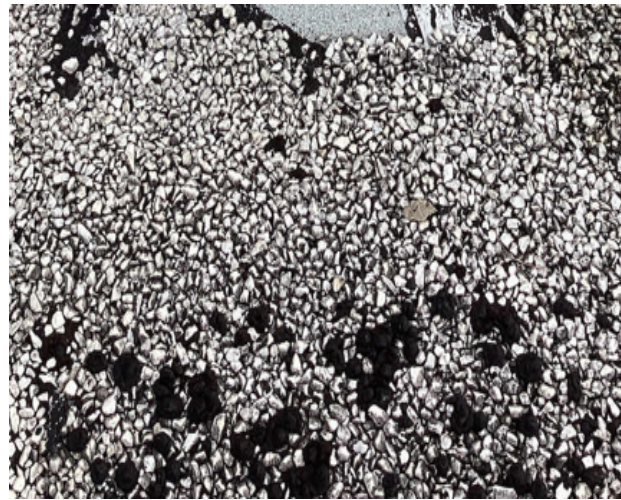
Flat Roof with Gravel Finish
