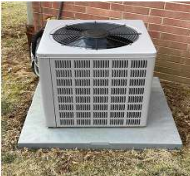
Exterior Condensing Unit
