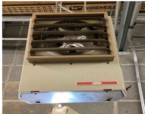
Elevated Electric Resistance Unit Heater
