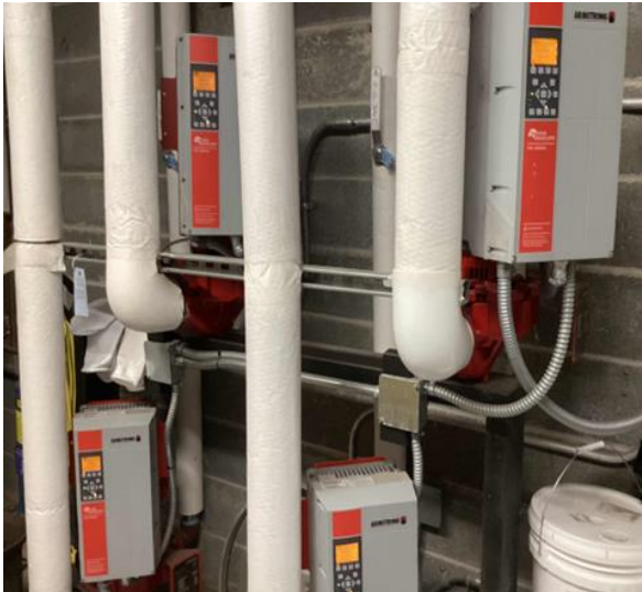
Four HHW Pumps with VFDs
