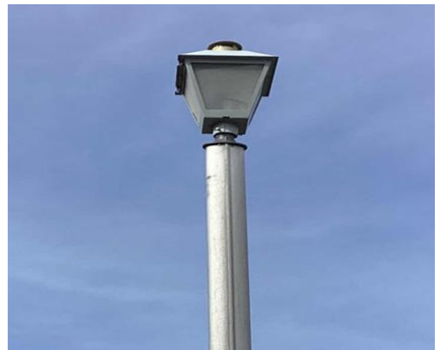
Pole Fixture with LED Bulb
