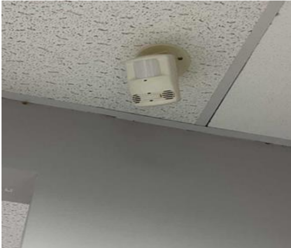
Ceiling Mounted Occupancy Sensor
