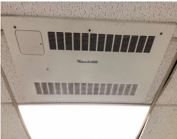
Ceiling Mounted Electric Resistance Heater
