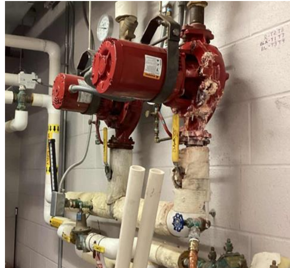
Two Constant Speed HHW Pumps
