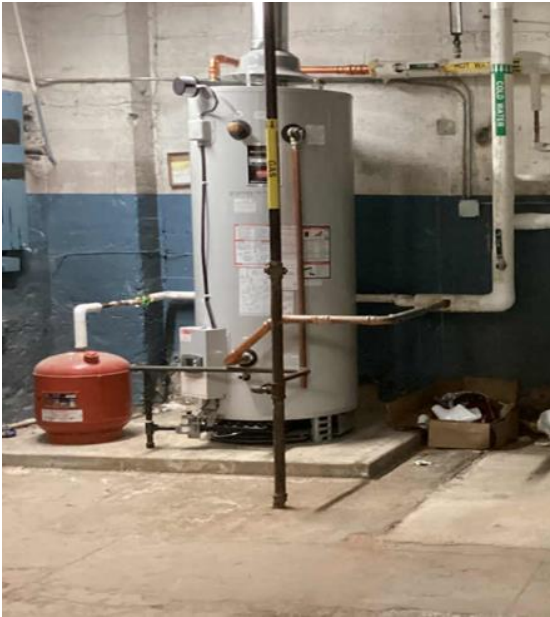
Gas-Fired Hot Water Heater
