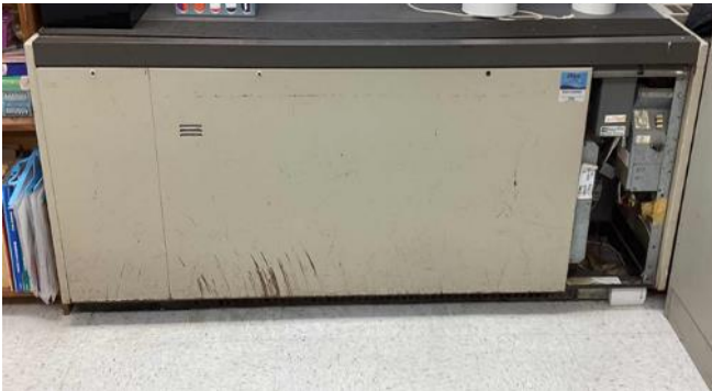
Typical Classroom Unit Ventilator
