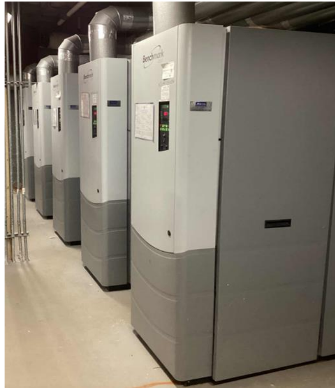
Condensing Boilers
