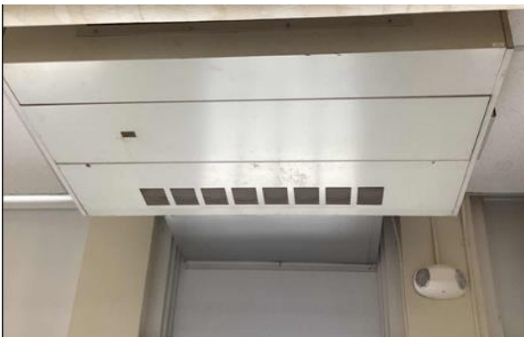
Electric Resistance Heat
