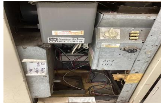
Typical Classroom Unit Ventilator
