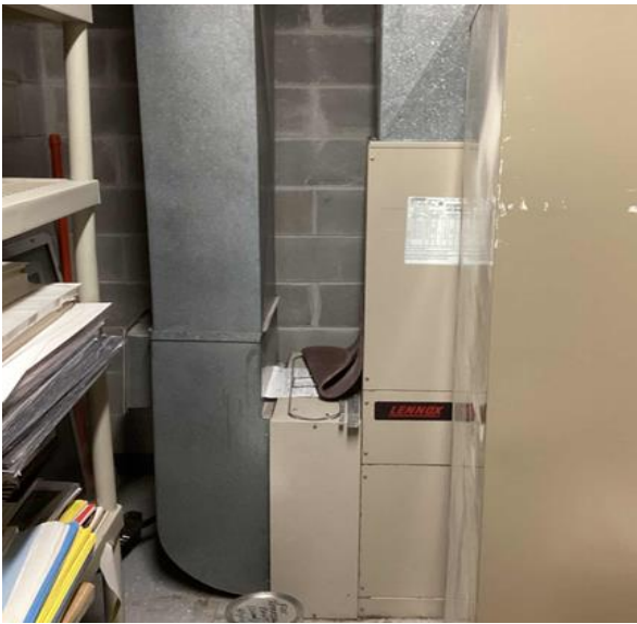
Electric Forced Air Furnace
