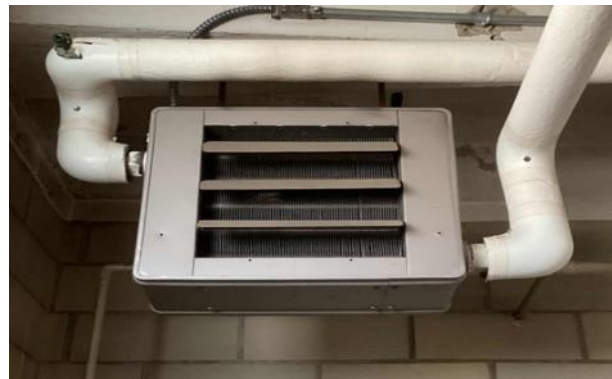
Suspended Hydronic Unit Heater
