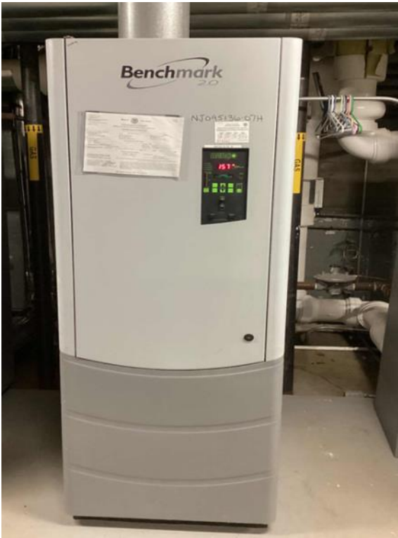
Condensing Boilers
