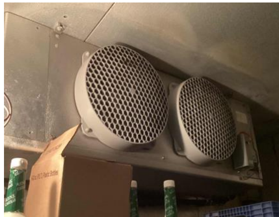
Two Fan Evaporator
