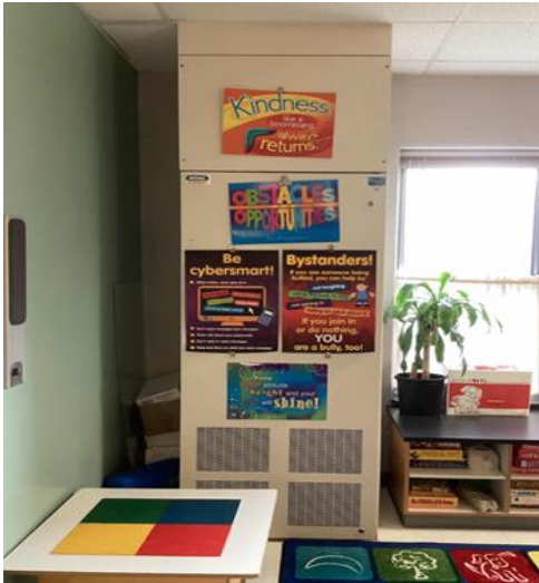
Vertical Unit Ventilator
