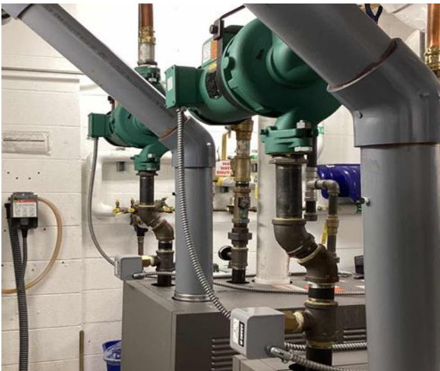
Heating Hot Water Pumps
