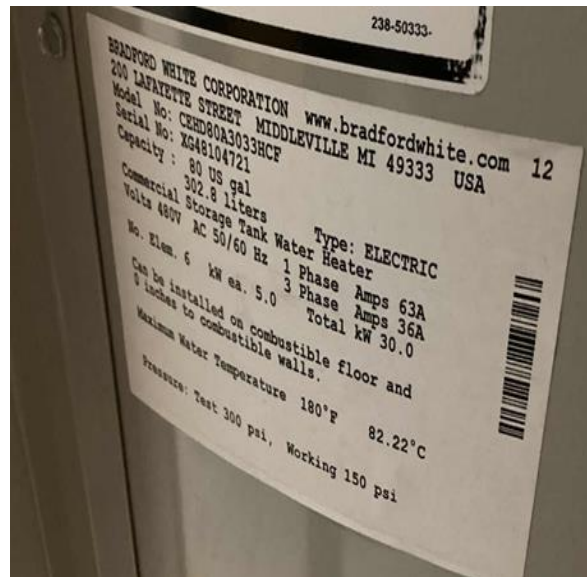
Electric Domestic Water Heater
