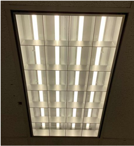
4 Foot LED Linear Tubes
