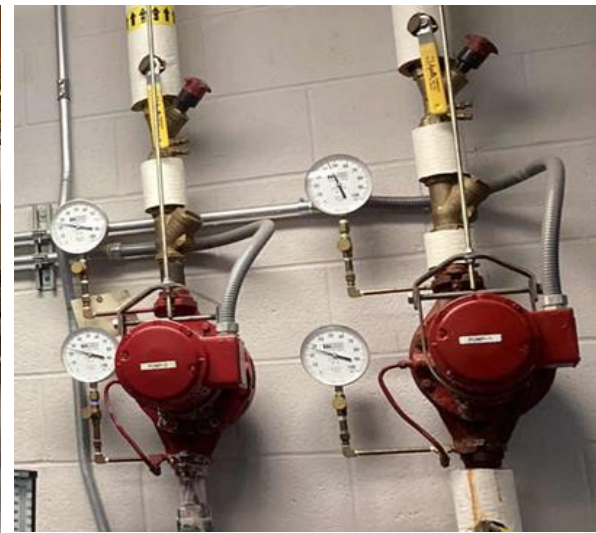
Heating Hot Water Pumps
