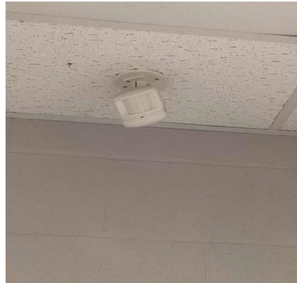
Ceiling Mounted Occupancy Sensor
