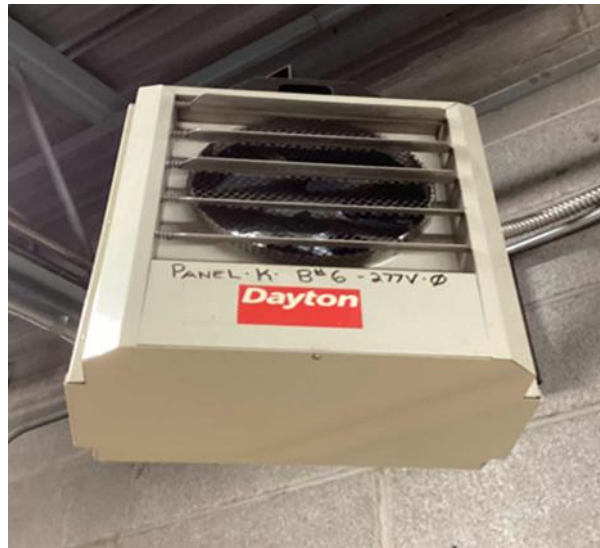
Elevated Electric Resistance Heater
