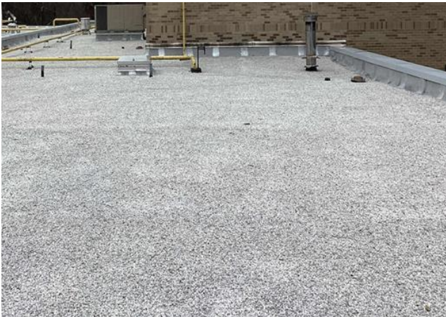
Flat Roof with Gravel
