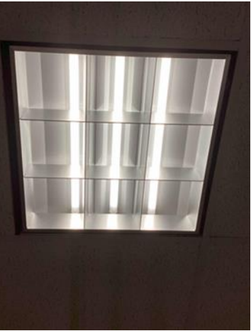
2 Foot LED Linear Tubes
