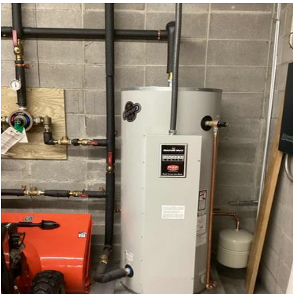
Electric Domestic Water Heater
