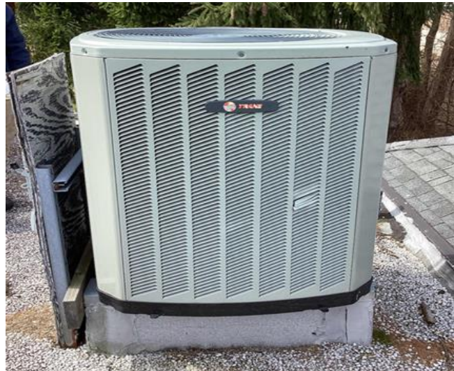
Split Air Source Heat Pump
