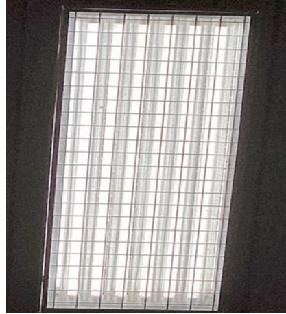
4 Foot LED Linear Tubes
