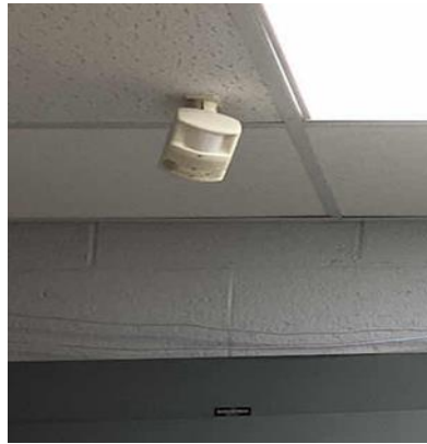
Ceiling Mounted Occupancy Sensor
