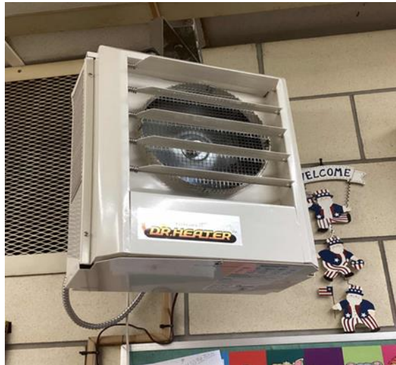
Electric Resistance Unit Heater
