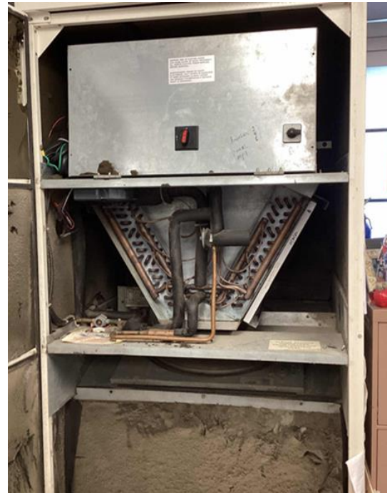
Airedale – Vertical Unit Ventilator
