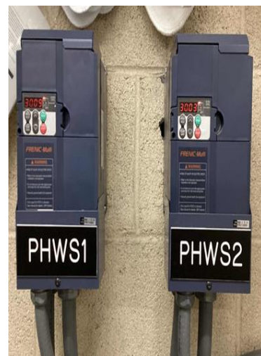
FDs for 7.5 hp Hot Water Pumps
