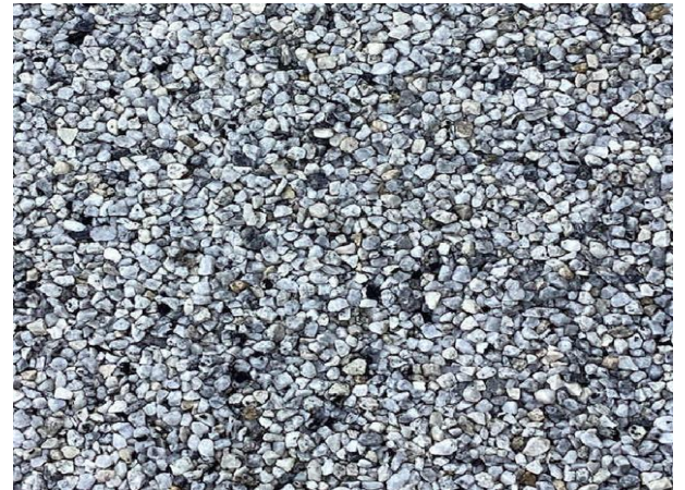
Flat Roof with Gravel Finish
