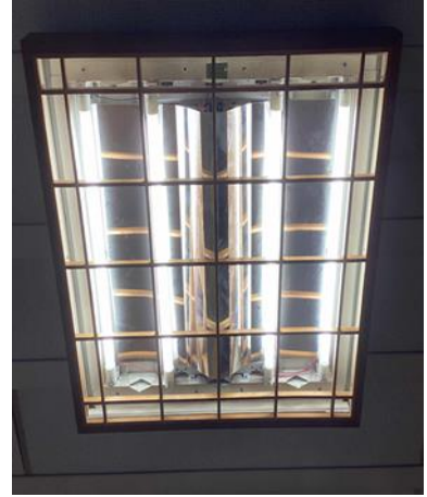
2 Foot LED Linear Tubes
