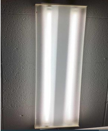
4 Foot Linear T8 Fluorescent Tubes
