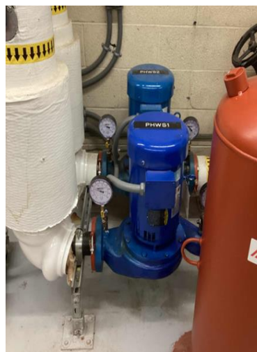
Two 7.5 hp Hot Water Pumps
