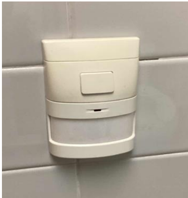
Wall Mounted Occupancy Sensor
