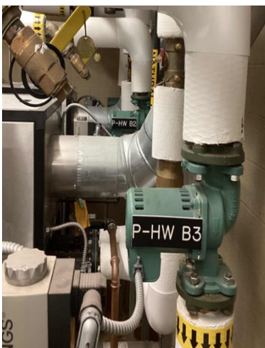
Three 0.5 hp Hot Water Pumps
