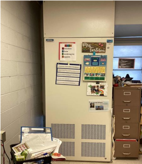
Airedale – Vertical Unit Ventilator
