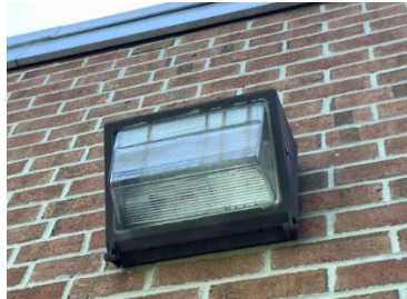
Courtyard – Metal Halide Fixture
