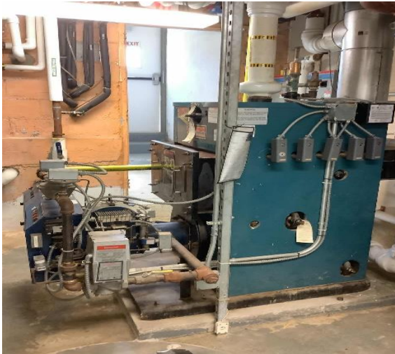
Burnham Boiler - 1921 Section
