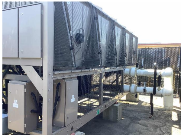
Air-Cooled Scroll Chiller
