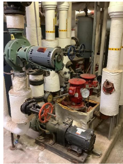
Heating Hot Water Pumps – 1965 Section
