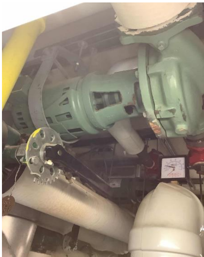
Heating Hot Water Pumps – 1921 Section
