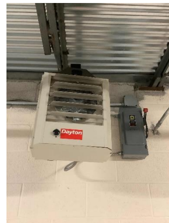
Electric Resistance Heater – Storage 1921 Section
