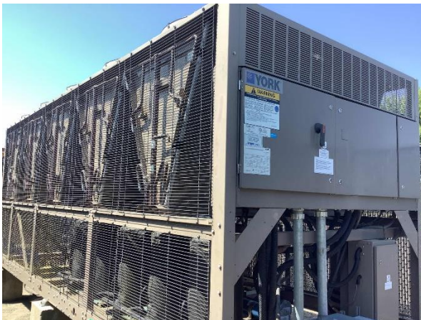
Air-Cooled Scroll Chiller
