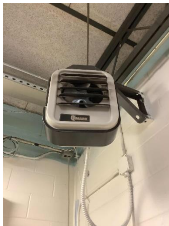
Electric Resistance Heater – Maintenance Shop
