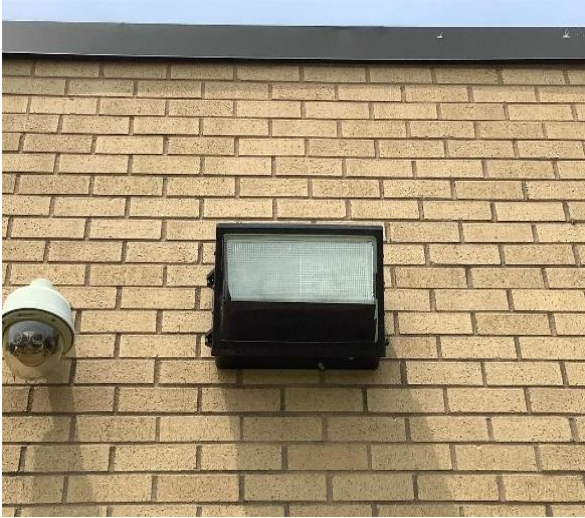
Exterior Wall Pack Fixtures
