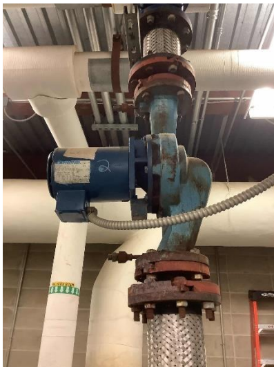
Heating hot water pump
