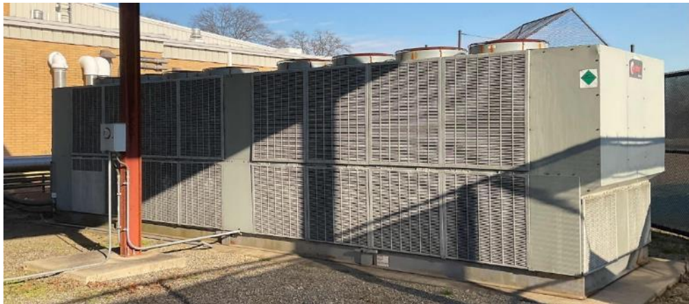
Trane air-cooled screw chiller
