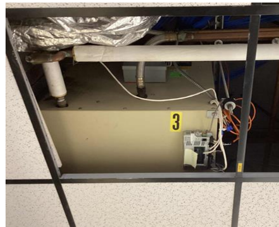
Above Ceiling Mounted WSHP
