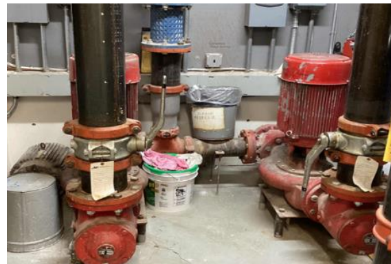
15 hp Water Circulation Pumps
