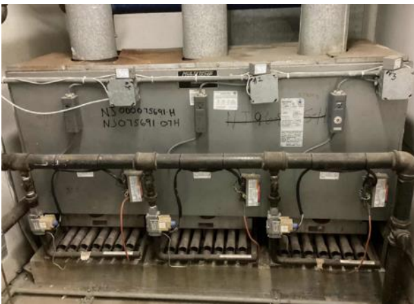
720 MBh Gas-Fired Boiler
