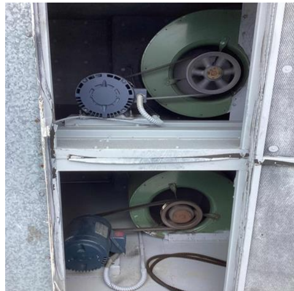
Supply and Return Fan Motors
