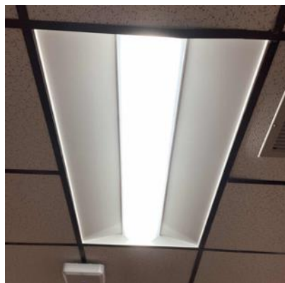
Linear T8 and LED Fixtures
