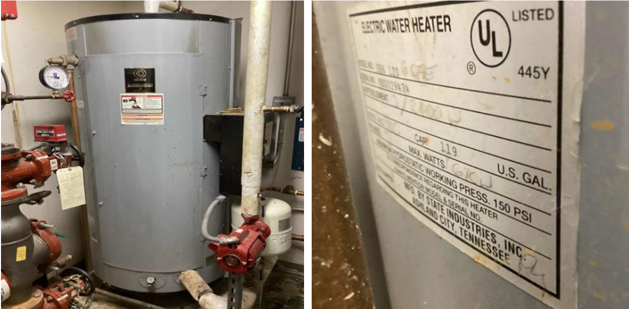
Electric Domestic Hot Water Heater
