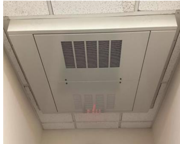
Ceiling Mounted Electric Resistance Heaters
