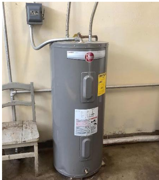
Storage Tank Water Heater
