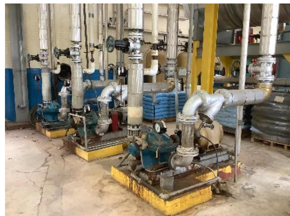
Boiler Feed Water Pump
