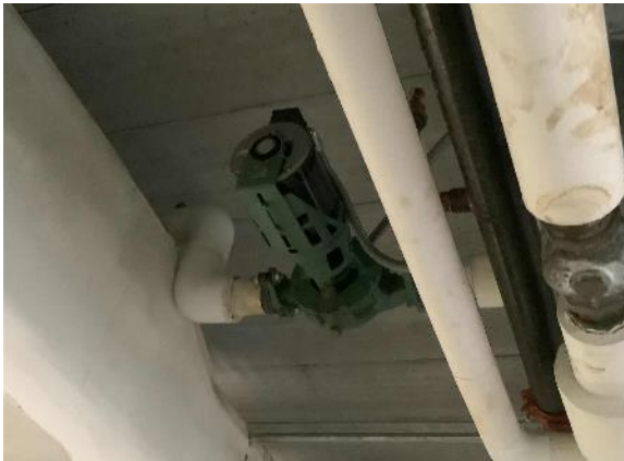
Hot Water Pumps- Roof Top Units
