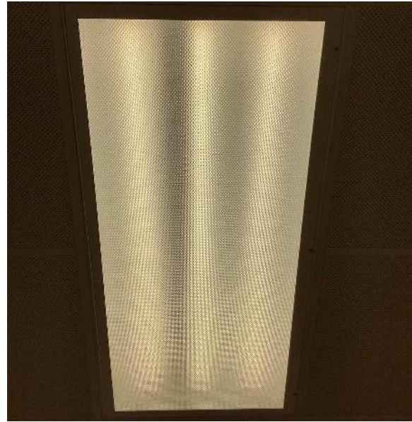
Linear Fluorescent T8 Lamps
