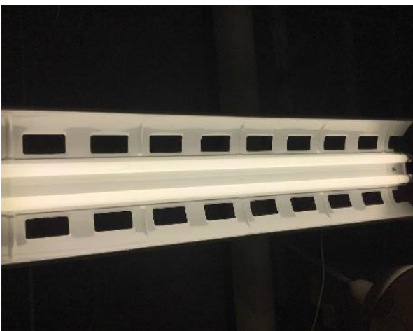
Linear Fluorescent T8 Lamps
