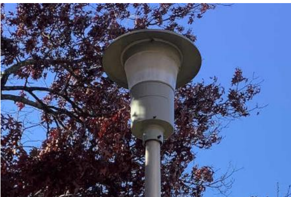
Exterior HID Pole Fixture
