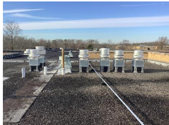
Roof: Exhaust Fans
