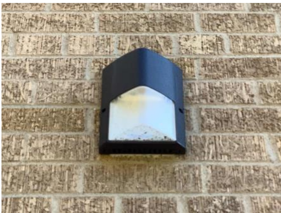
Exterior LED Wall Pack Fixture
