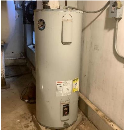
Electric Storage Tank Water Heater
