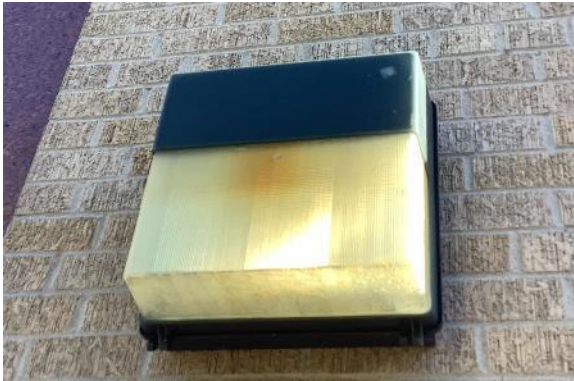
Exterior HID Wall Pack Fixture
