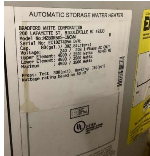
DHW Tank Water Heater Nameplate
