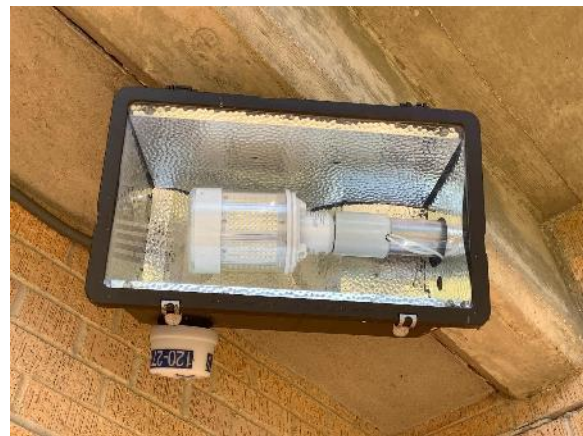
Exterior LED Corn Bulb Fixture
