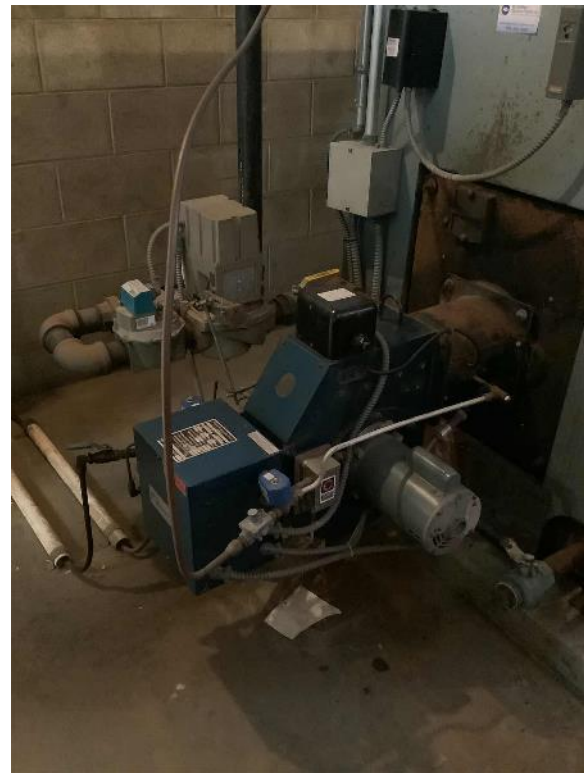
Boiler Combustion Fan: Greenhouse
