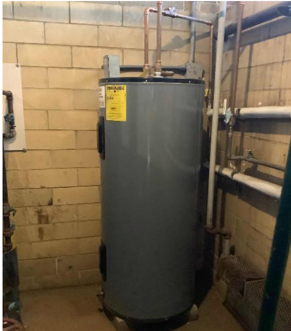
Electric Tank Storage Heater: Greenhouse
