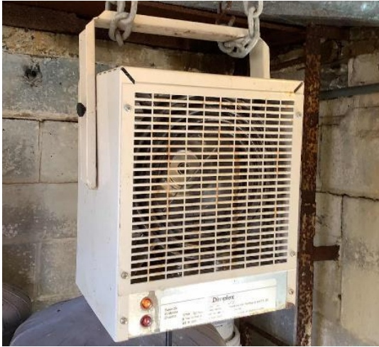
Electric Resistance Heater: Pool House
