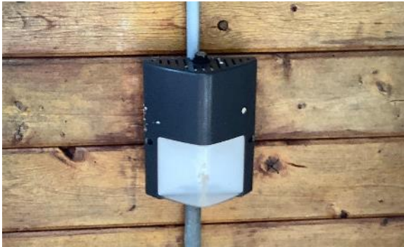
Exterior LED Wall Pack: Greenhouse
