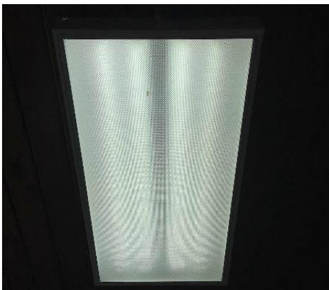
Linear Fluorescent T8 Lamps: Greenhouse
