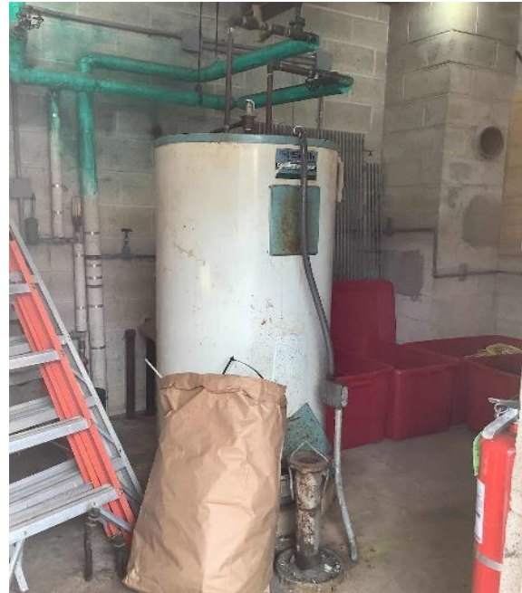
Electric Tank Storage Heater: Pool House
