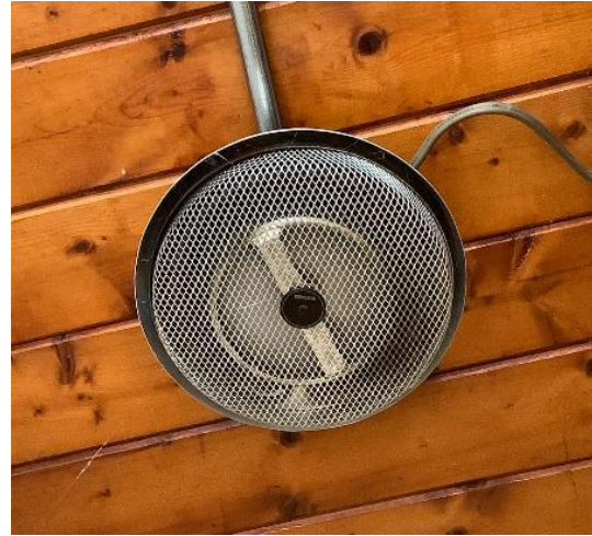
Electric Resistance Heater: Pool House
