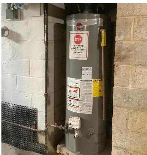
Gas-Fired Storage Tank Water Heater: 60 Laurel Lane
