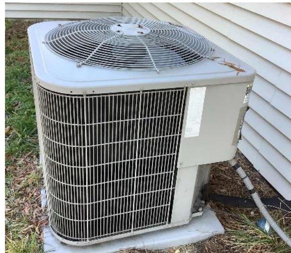
Typical Outdoor Condensing Units
