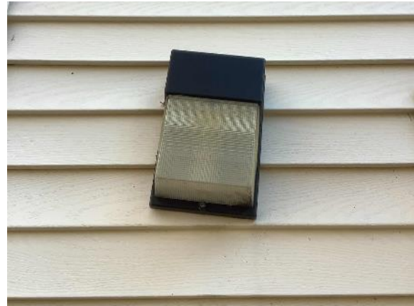
Typical Exterior CFL Wall Pack Fixture
