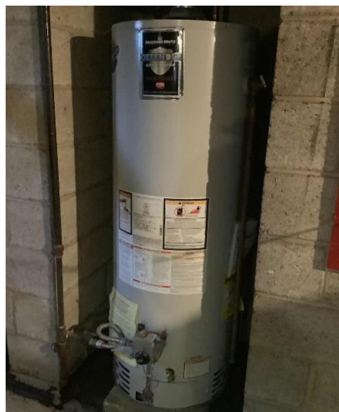
Gas-Fired Storage Tank Water Heater: 46 Fern Lane
