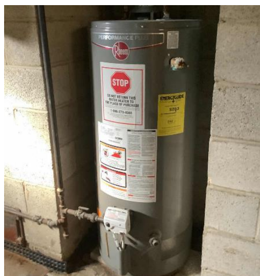
Gas-Fired Storage Tank Water Heater: 44 Fern Lane
