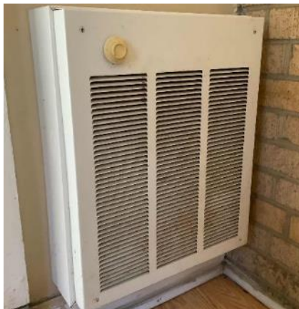
Electric Resistance Heater-41 Fern Lane
