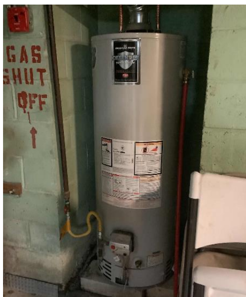
Gas-Fired Storage Tank Water Heater: 41 Fern Lane
