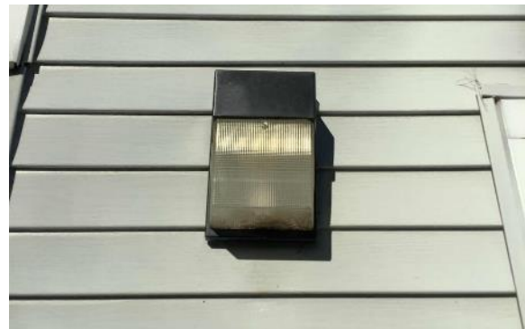
Typical Exterior CFL Wall Pack Fixture
