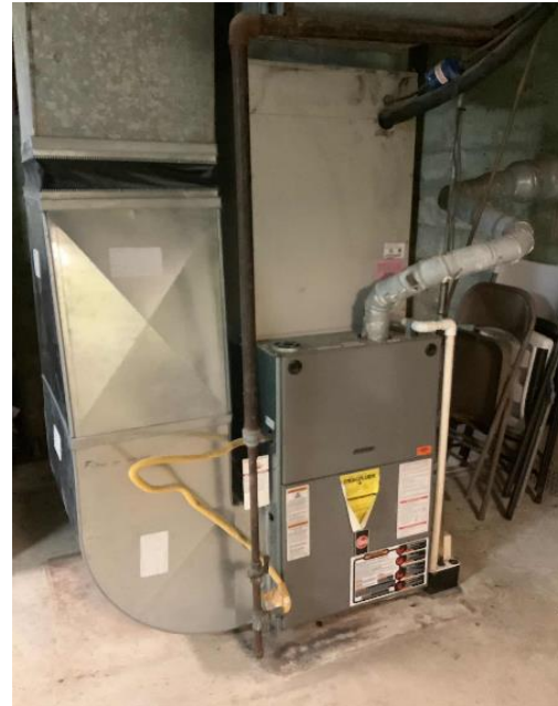
Gas-Fired-Heating Furnace
